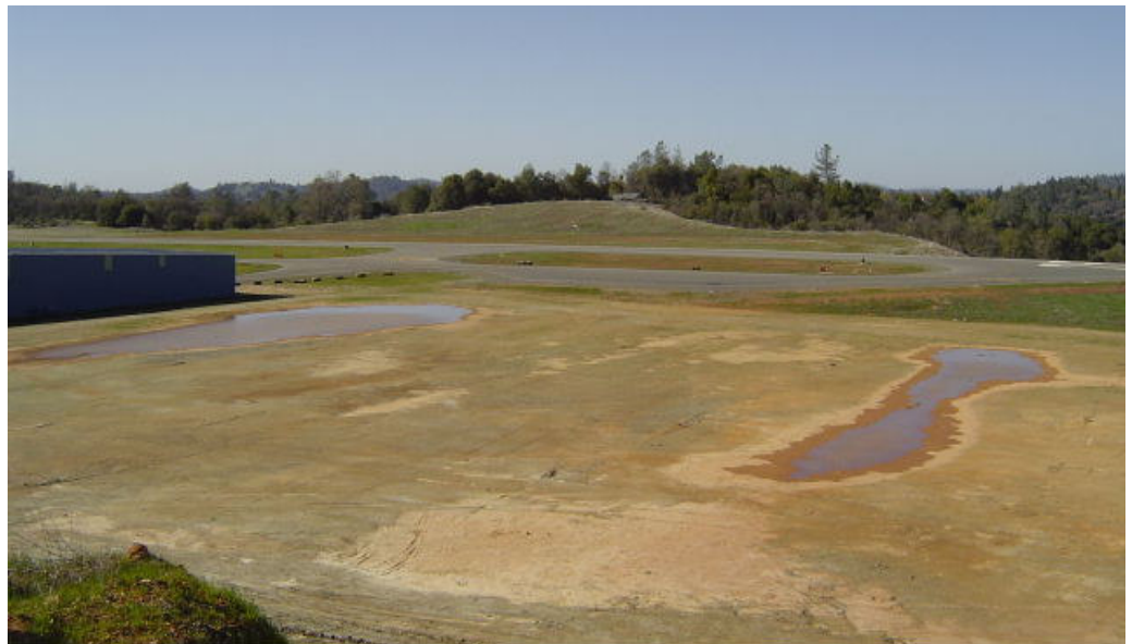
East Hanger Project as it looked on March 12th 2004
